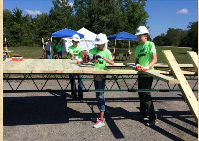
Using a power drill to create decking
